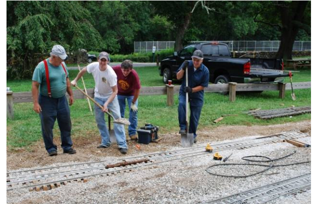
Helping To Install the South Station Switch
