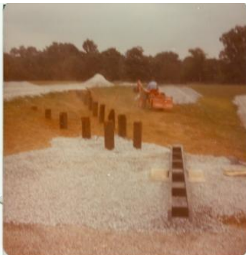
Left: Working on lead from yard to lift. Air compressor used before Midway was built.
