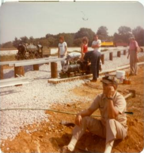
Left: Now have first bay track installed.
