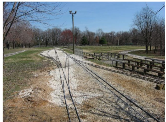
(6) New Switch – Connector Does Wriggle
