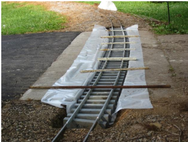
(3) Track Suspended for Concrete Base
