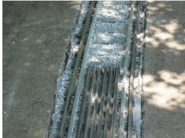
(4) Rails Inside & Out Provide Vehicle Crossing
